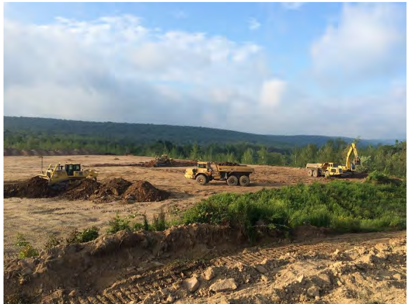
KT Holdings Site Construction
